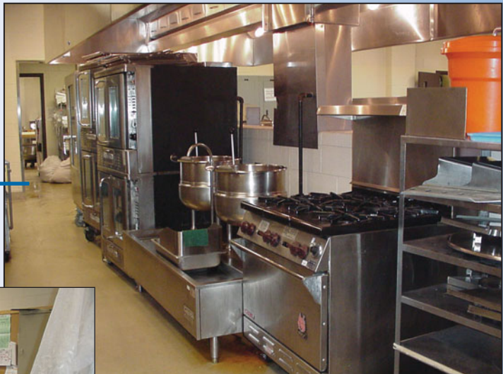
Production equipment: combi-ovens, trunnions, and a range
