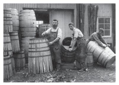
Several of the barrels on the left side of this 19th-century photo have not been fired to curve their staves. The cooper on the left is shown with his hammer and hoop driver. The one in the centre is planing the croze to accept a head, and one on the right, an apprentice, is shaving the outside to clean the barrel, a finishing procedure.
